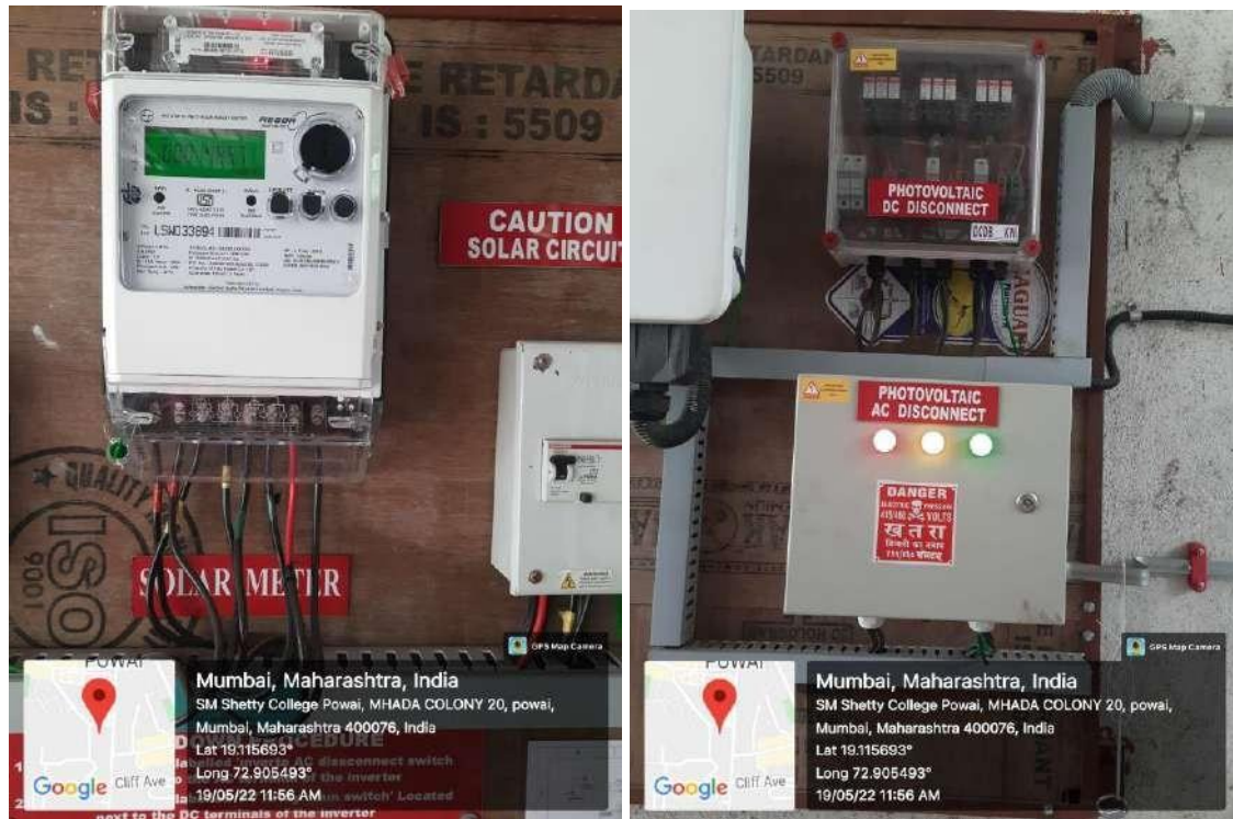
Netmeter for accessing solar energy generated
