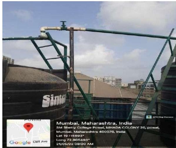
BMC water inlet for both drinking water tanks and multi-purpose tanks
