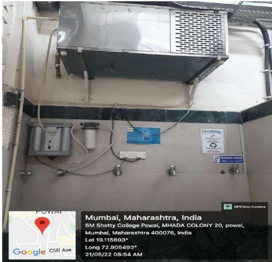
Water purifying and cooling systems installed on every floor ( four in total)
