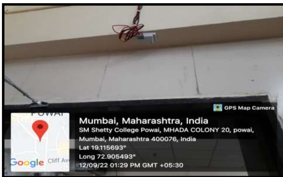
Staff washroom have been installed with motion based light sensors
