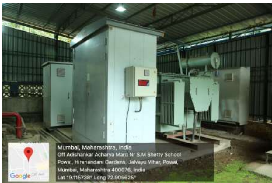
Power Generation System of Solar Panel in the campus
